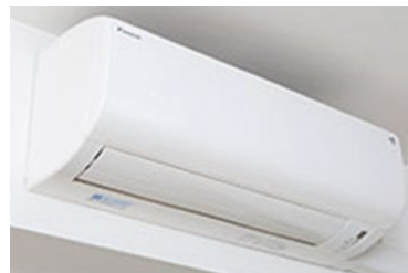
Replacing air conditioners
