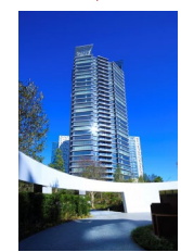
COMFORIA SHINJUKU EASTSIDE TOWER
